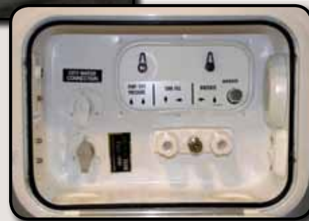
Exterior water center access.
